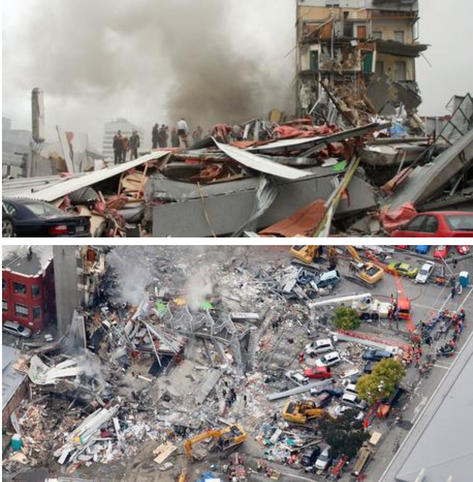
Collapse of the 5-story CTV building in Christchurch, New Zealand
